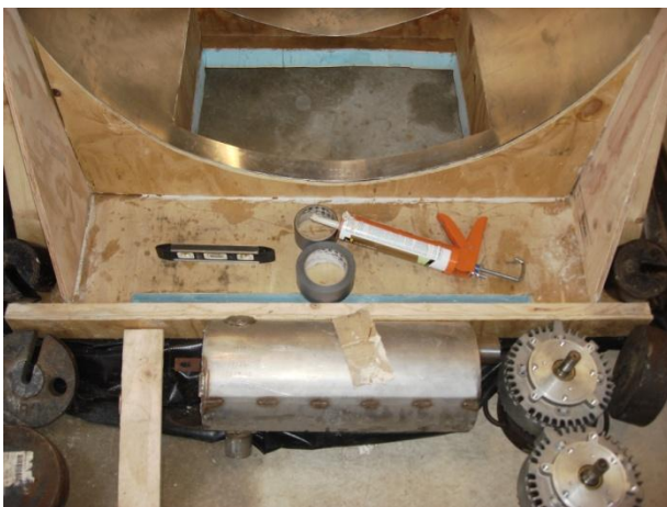
Figure 26: Construction of final air box design
