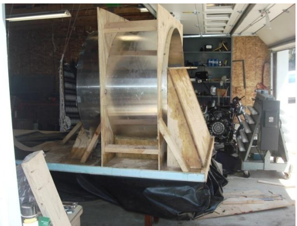
Figure 27: Side view of air box after construction
